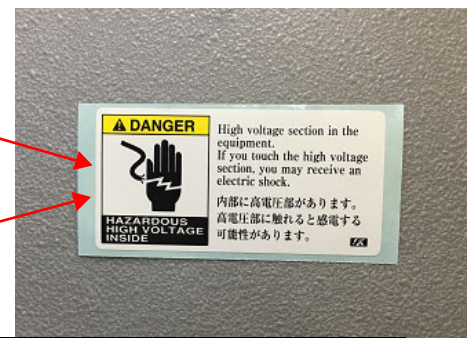
M903764_Caution label- UV power voltage
